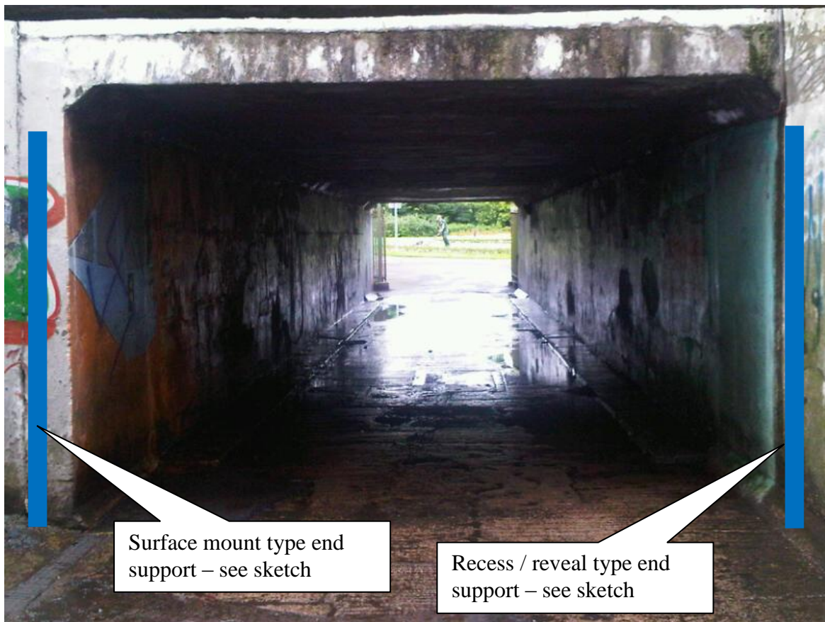
Photograph of end of underpass with end supports indicated
