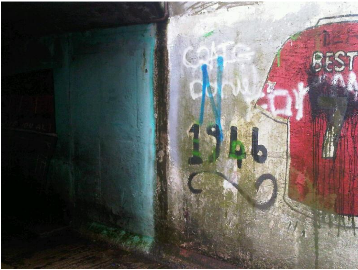
Further photos of underpass sides
